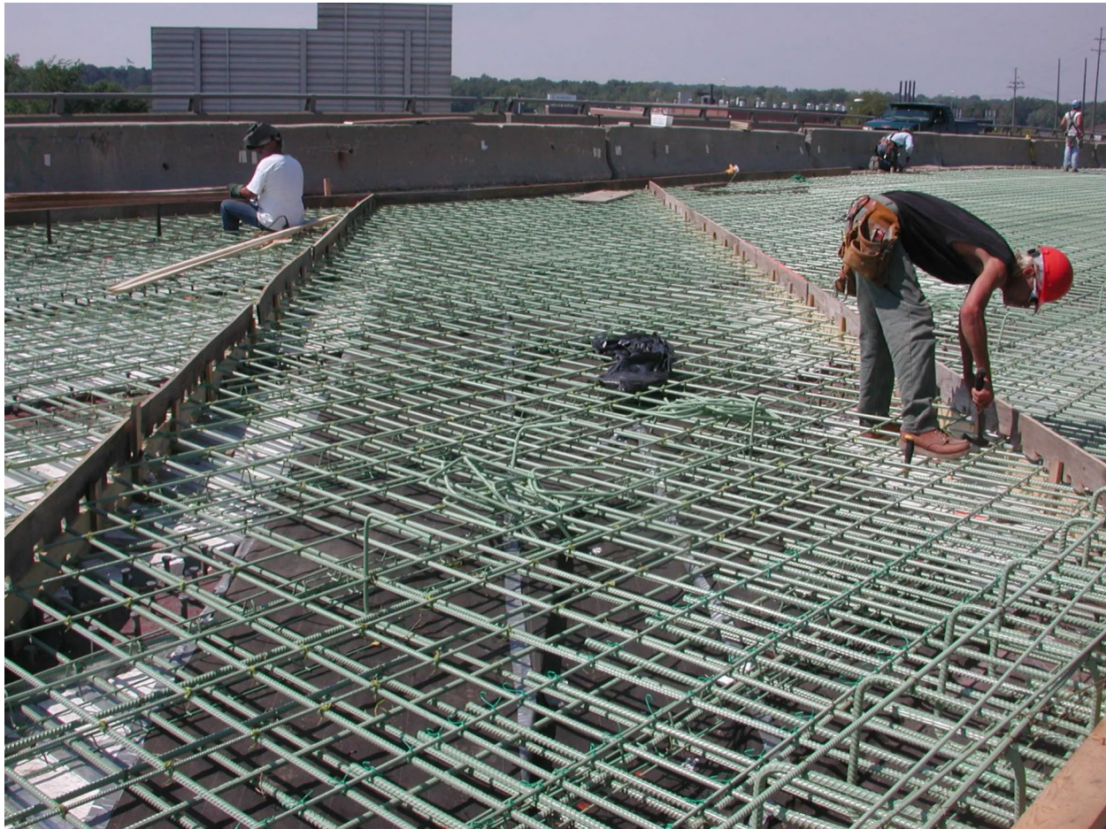
Fig. 4 Traditional construction site: The placing of reinforcements
