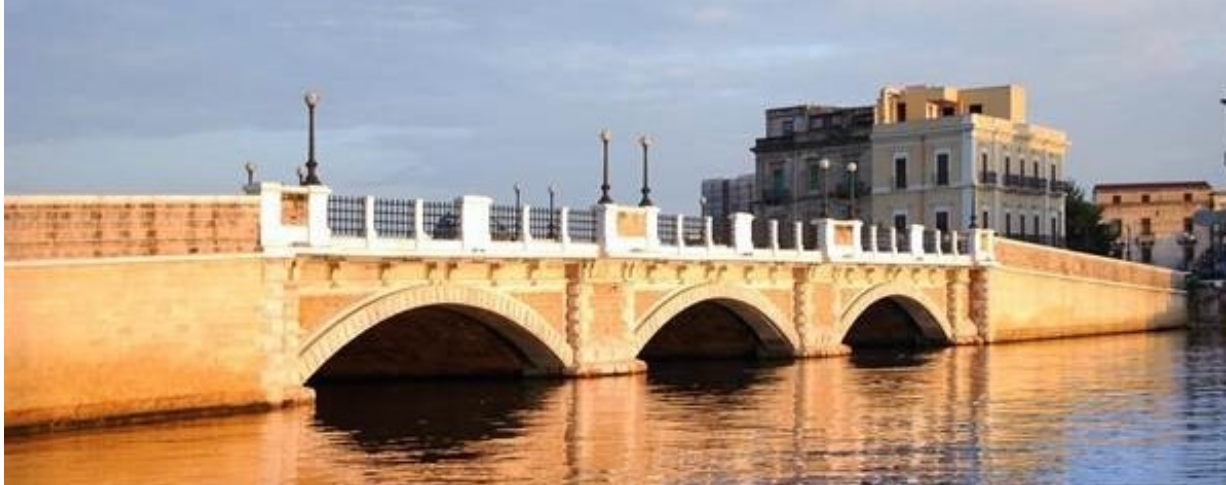
Figure 2: Porta Napoli bridge. View from Mar Piccolo.
